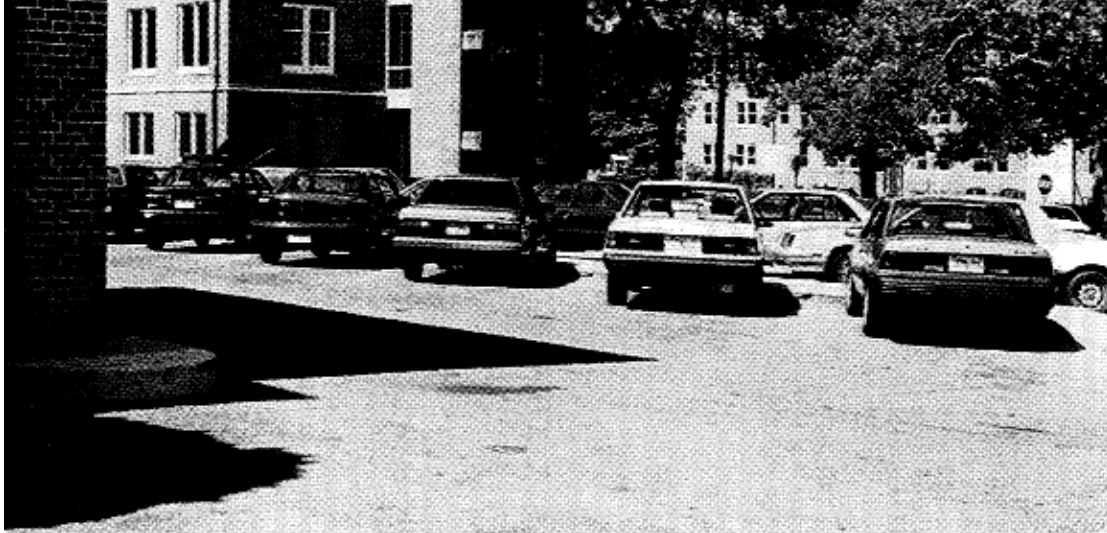
Photo 16.5 Parking; Typical Small Asphalt Paved Lot
