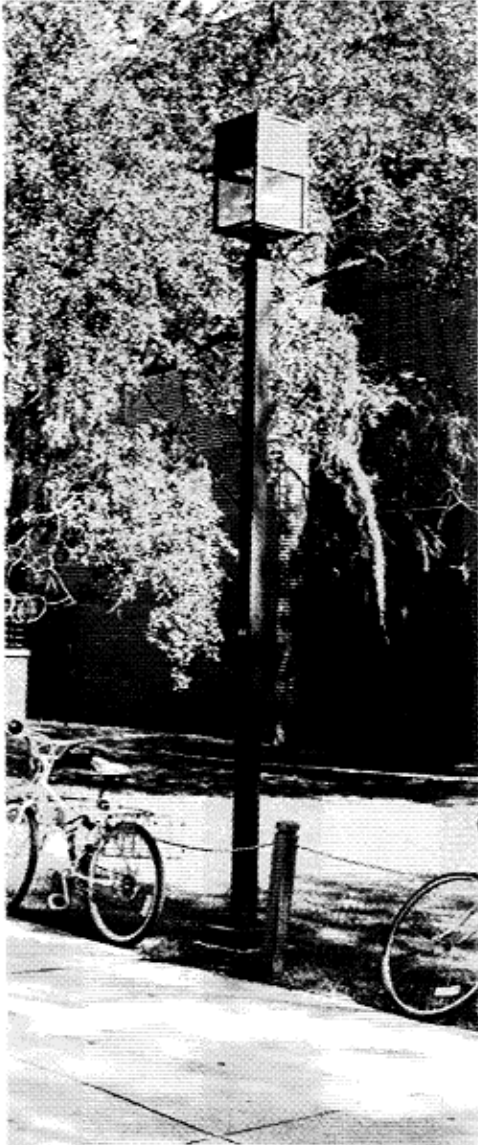
C. Metal Fixture And Pole
